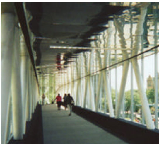
The Underground Walk went to the Plaza of the Americas (above) and through one of several sky bridges (below).
